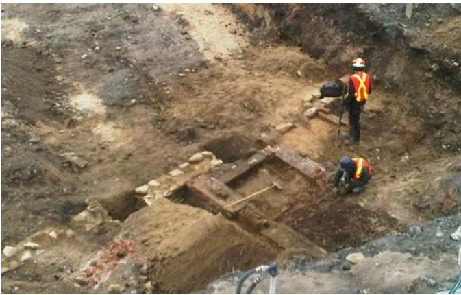
Archaeologists at work on the site of Context Development's new project at the foot of Bathurst Street
